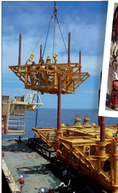
For the Cascade-Chinook subsea hardware installation program in the deepwater Gulf of Mexico, Technip's Deep Blue used lifting slings (inset) fabricated by SWOS using Samson's AmSteel-Blue rope.
